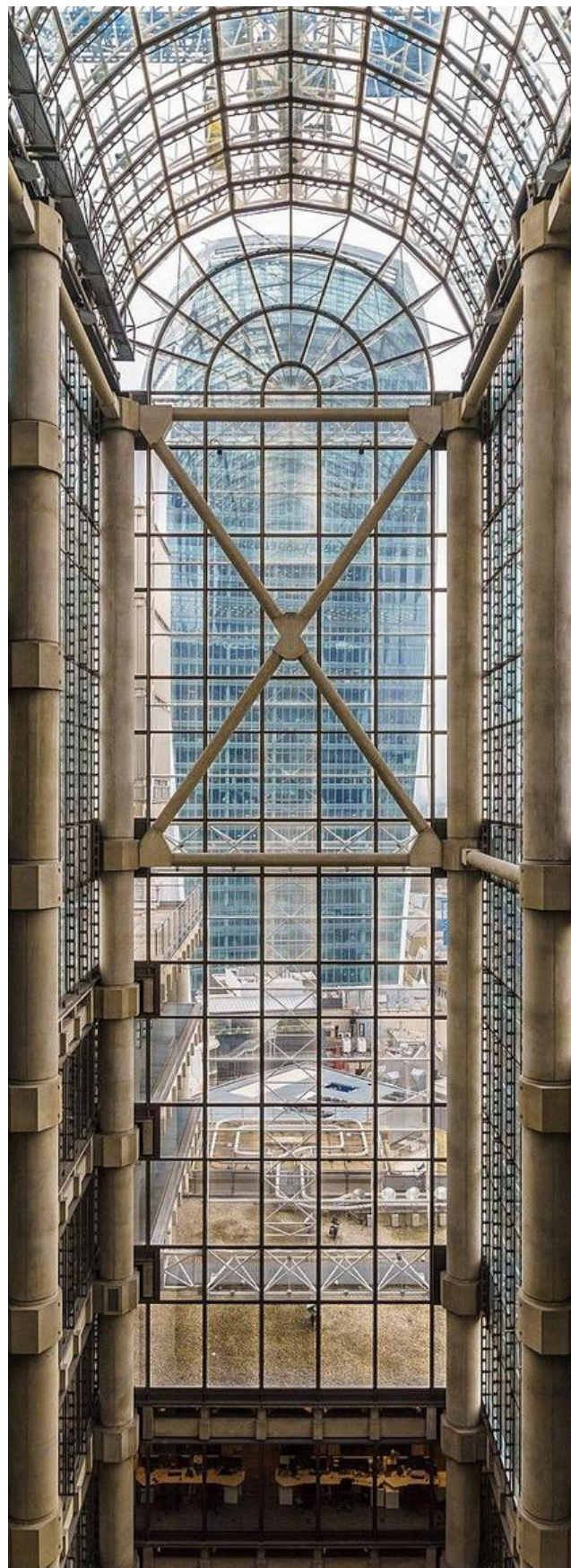
Vertical window of the Lloyd's Building
