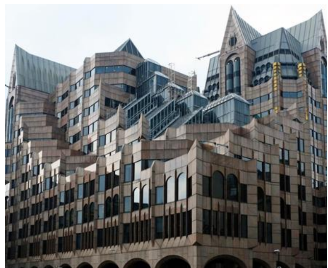
Minster Court building
