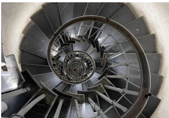
Spiral staircase Monument to the Great Fire
